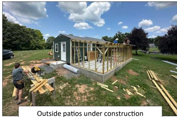
Outside patios under construction
